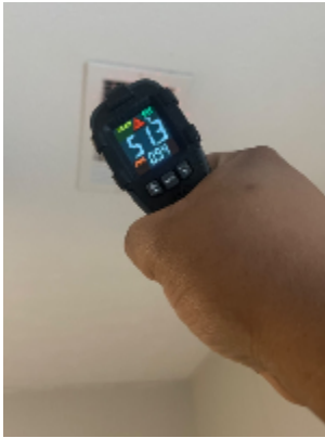
Cold air temp reading
